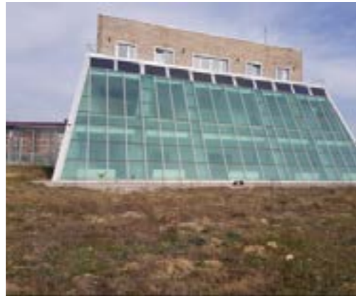
Figure 2.3 Façade Mounted Solar Panels at Gökçöy Campus
